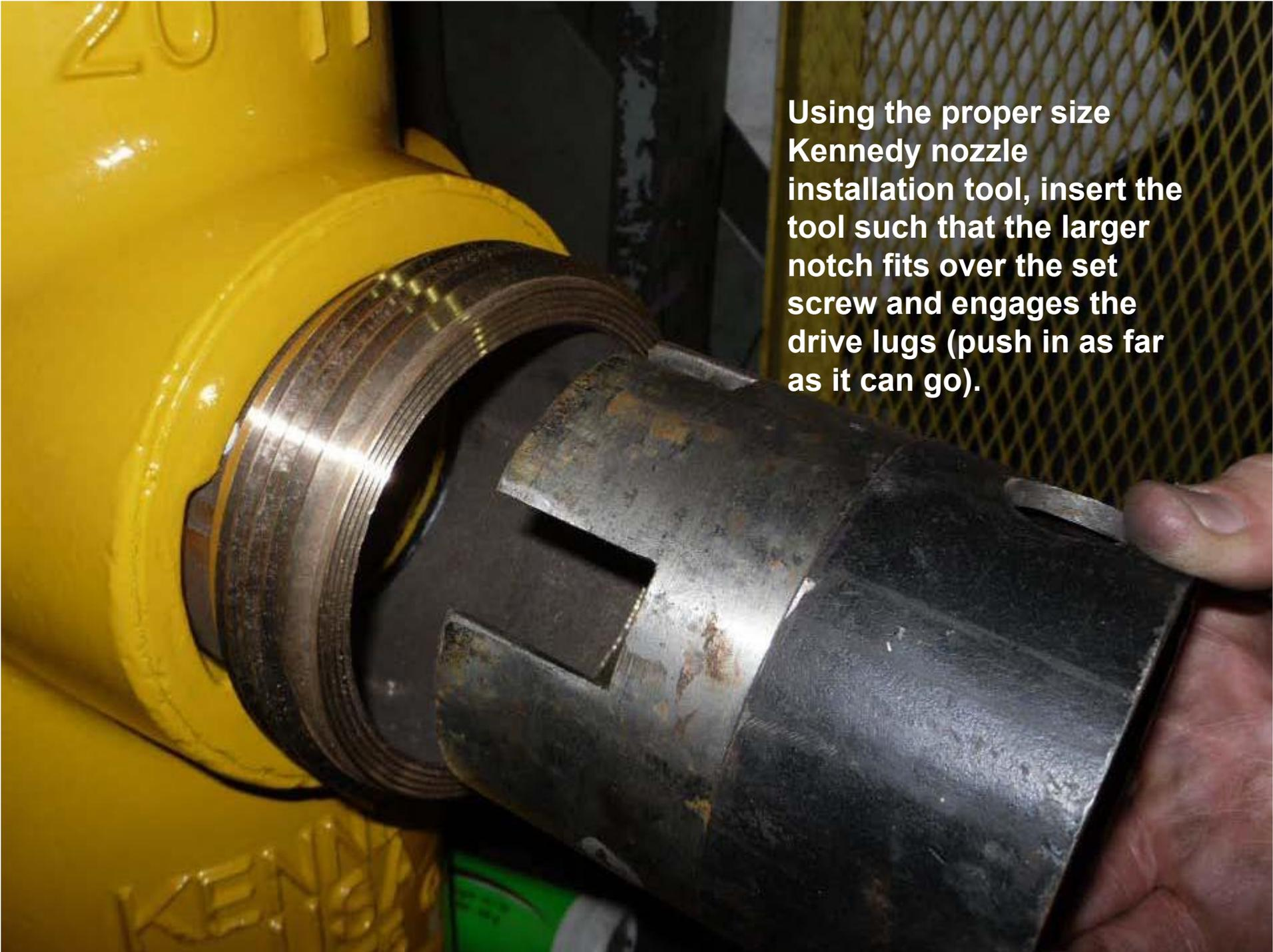
Using the proper size Kennedy nozzle installation tool, insert the tool such that the larger notch fits over the set screw and engages the drive lugs (push in as far as it can go).
