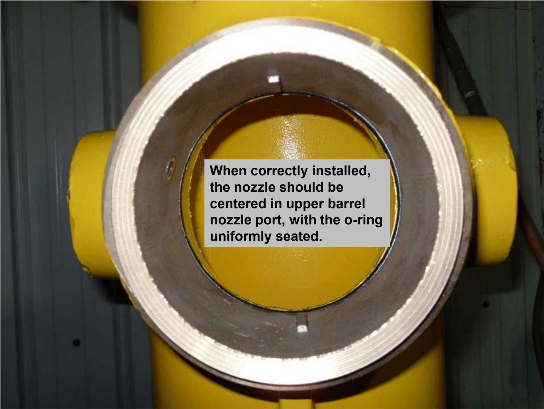
**When correctly installed, the nozzle should be centered in upper barrel nozzle port, with the o-ring uniformly seated.**
