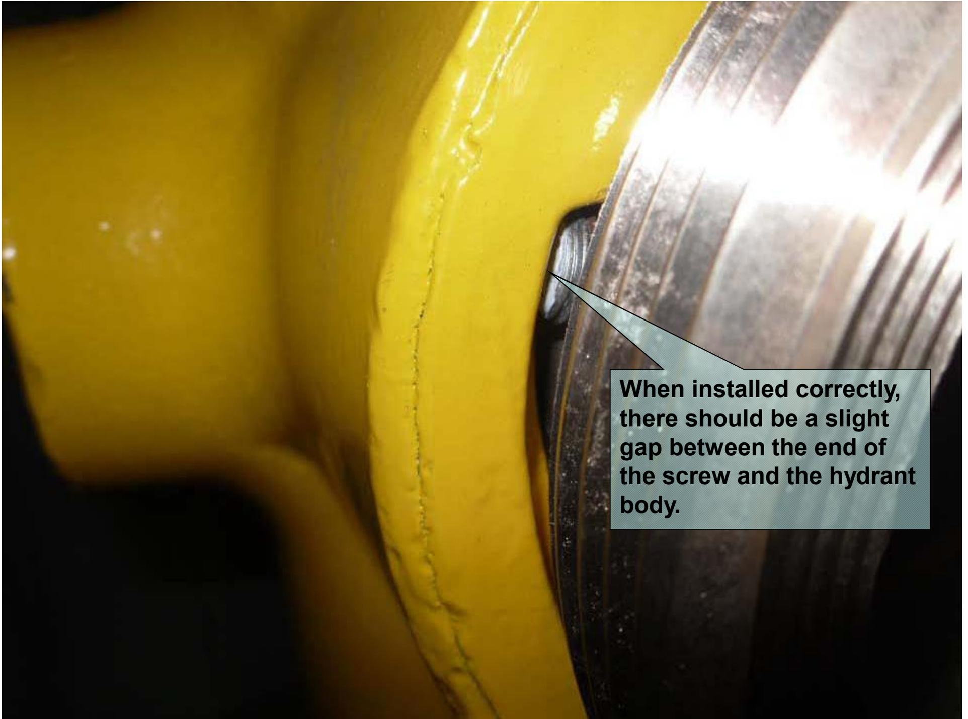
**When installed correctly, there should be a slight gap between the end of the screw and the hydrant body.**
